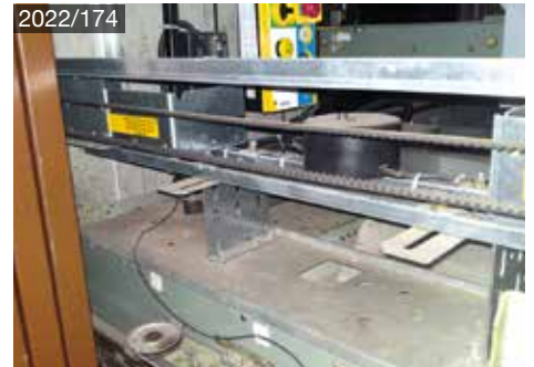
Otis GMP telescope
