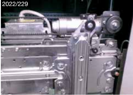
Selcom Mosquito telescope
