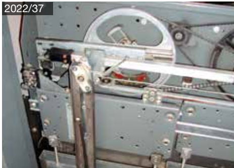
Fermator Sinus telescope
