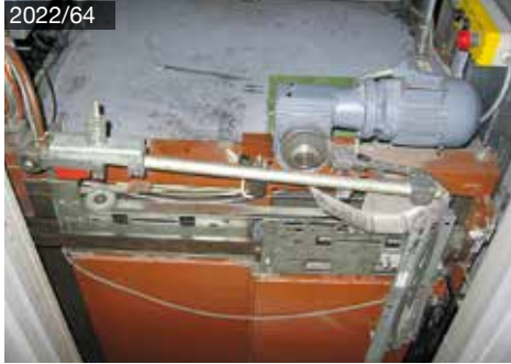
Haushahn TASS80 telescope
