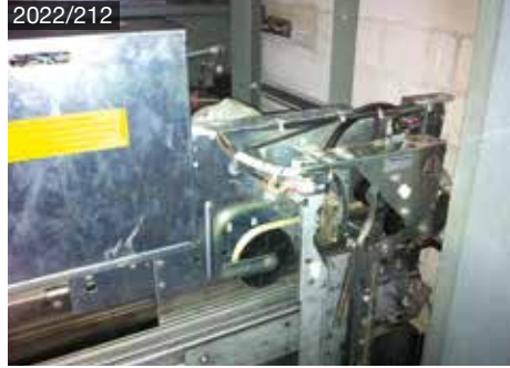
Schindler QKS11 telescope
