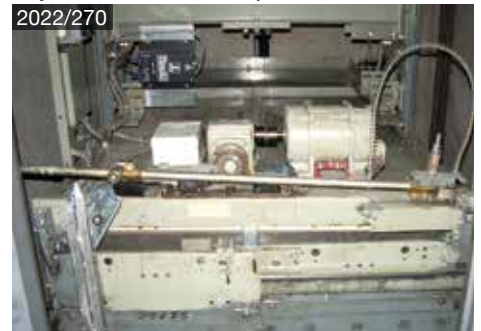
Thyssen M2T D4 telescope
