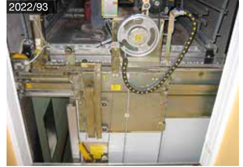
Kone ADC telescope
