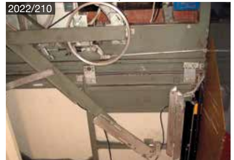
Schindler QKS9 telescope
