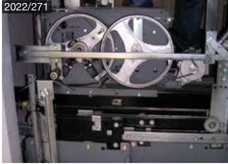
Thyssen M2T D6 telescope
