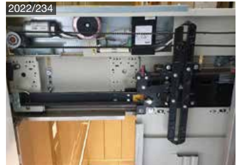
Sematic 2000 Code B105AANX telescope
